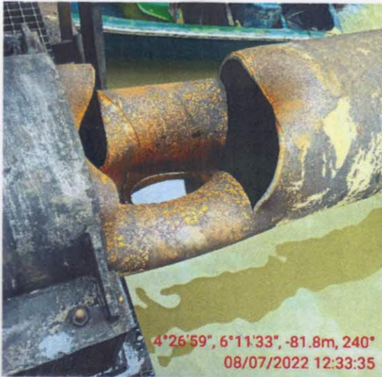
PICTURE A: SHOWING BLASTED PORTION OF THE RISER AT 12 O' CLOCK POSITION. PICTURE B: SHOWING REPAIRED SECTION OF THE RISER.
